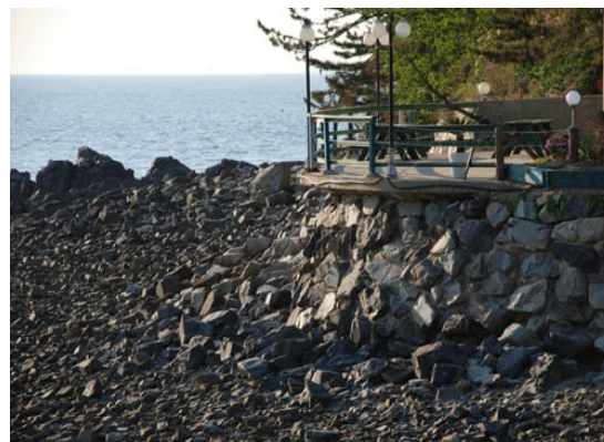
Fig. 16. Washed away Hardness shore protection (Mageom-po, 10. 2011).
