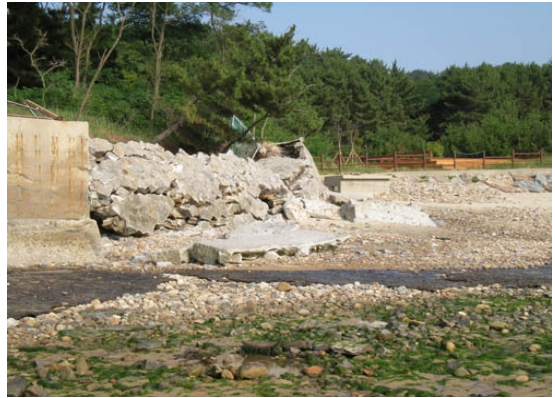
Fig. 19. Collapse of protective wall (Cheonri-po beach, 8. 2011).
