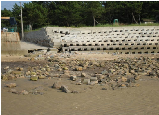
Fig. 18. Collapse of a gentle-slope hardness shore protection (Cheonri-po beach, 8. 2011).
