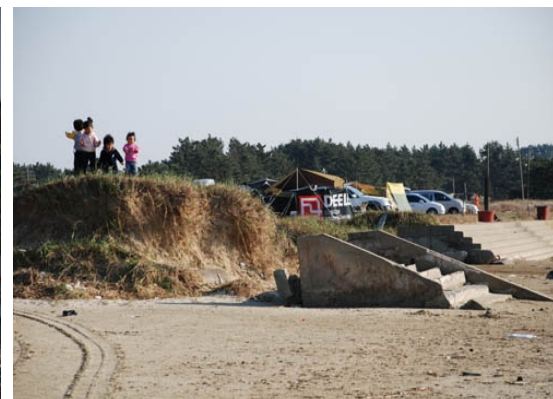
Fig. 17. Collapse of a gentle-slope hardness shore protection (northern part of Cheongpodae beach, 10. 2011).
